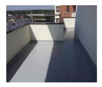
The Fatra liquid applied waterproofing system is a single component, unreinforced, polyurethane liquid waterproofing coating that contains a humidity activated technology to provide a highly elastic and hydrophobic membrane.
