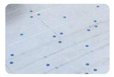
Insulation secured with FR-75 tube washers
