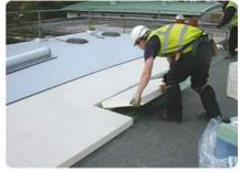
Positioning the insulation boards
