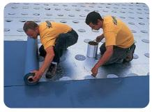
Lining up and rolling out the membrane
