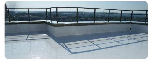
The system is a single component, unreinforced, polyurethane liquid waterproofing coating that contains humidity activated accelerator technology to provide a highly elastic and hydrophobic membrane. Due to the unique formulation, the Fatra liquid system cures to form a completely defect free membrane with excellent mechanical and elastomeric properties, high tensile & tear strength and exceptional adhesion properties.
