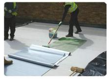
Applying FF859 adhesive to the insulation
