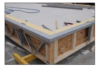
The above picture illustrates the use of membrane coated metal angles (to which the membrane can be easily welded), pre-formed corners, fixings and flashing membrane. All of these items are available from Fatra.
